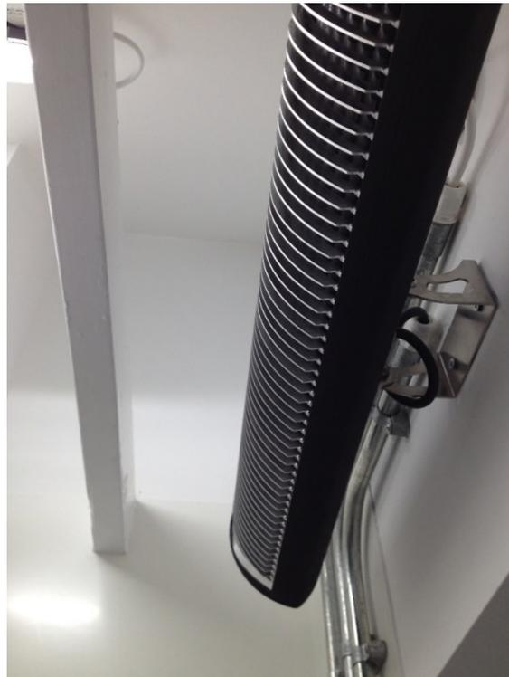
Manufacturer's instructions stated "Heater should be placed at least 750mm from any surface"
