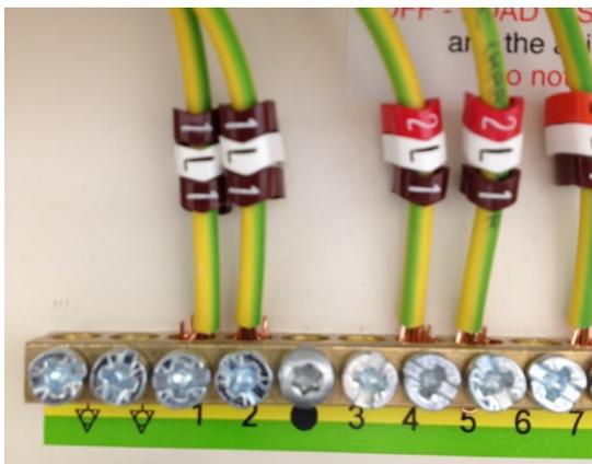
High integrity earthing, ring main cables to be in separate terminals.
