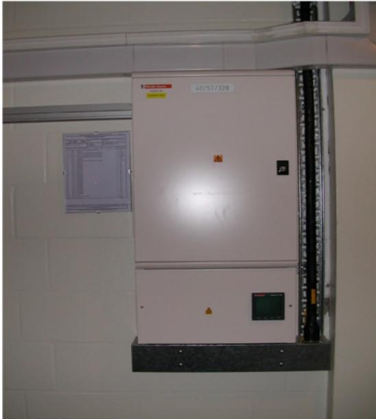
This is the University's preferred method of SWA cable installation into a Distribution board. This method complies with Code of Practice regarding live work whereby no live cables will be present in the distribution board when isolated locally
