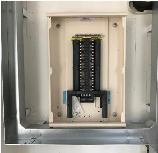
Distribution boards shall have 25% spare capacity at handover.
