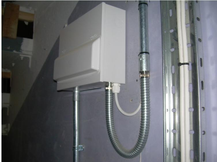
Kopex should be used in an appropriate manner i.e. for connections between isolators/plug and sockets and vibrating equip
