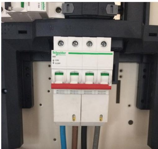
Cables supplying DB's should enter through bottom of DB. Cables should not pass through dis-board. 4 pole disconnecter is a requirement.
